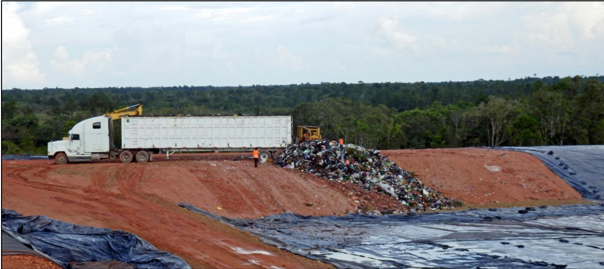
Figure 10: Bulk Transfer Vehicle Discharging MSW at Mile 24 Sanitary Landfill
