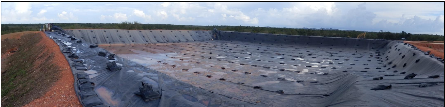
Figure 2: New Landfill Cell for Stabilised Hazardous Wastes at Mile 24
